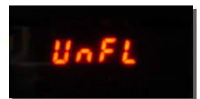
Under- and overflow indication
